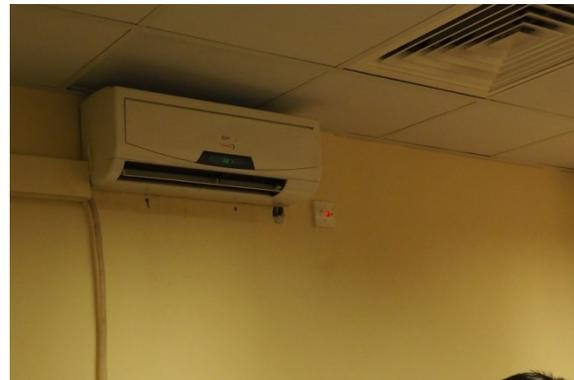
Figure 13: Freestanding climate unit next to a vent for the central climate system at the Ministry of Interior.
